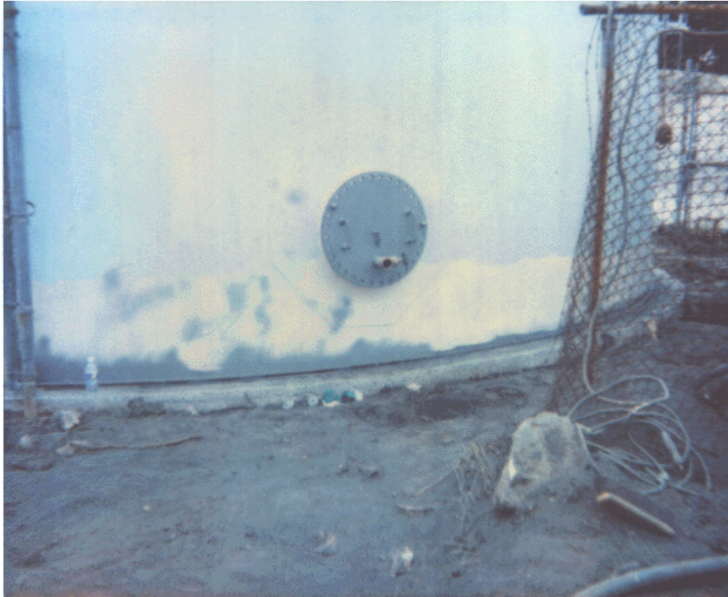
Picture of access / egress portal to water tank. The diameter of the access / egress is 24 inches and is 21 inches from the top of the concrete base, which is 5 inches deep.
