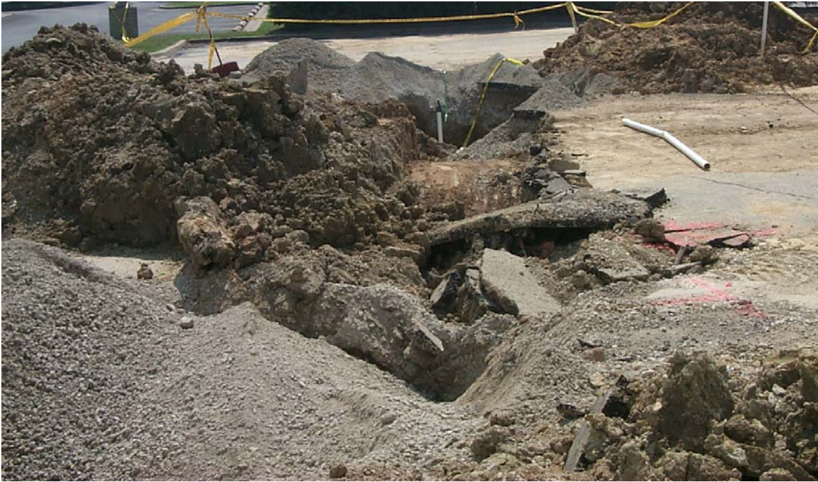
Excavation site where waterline was being repaired
