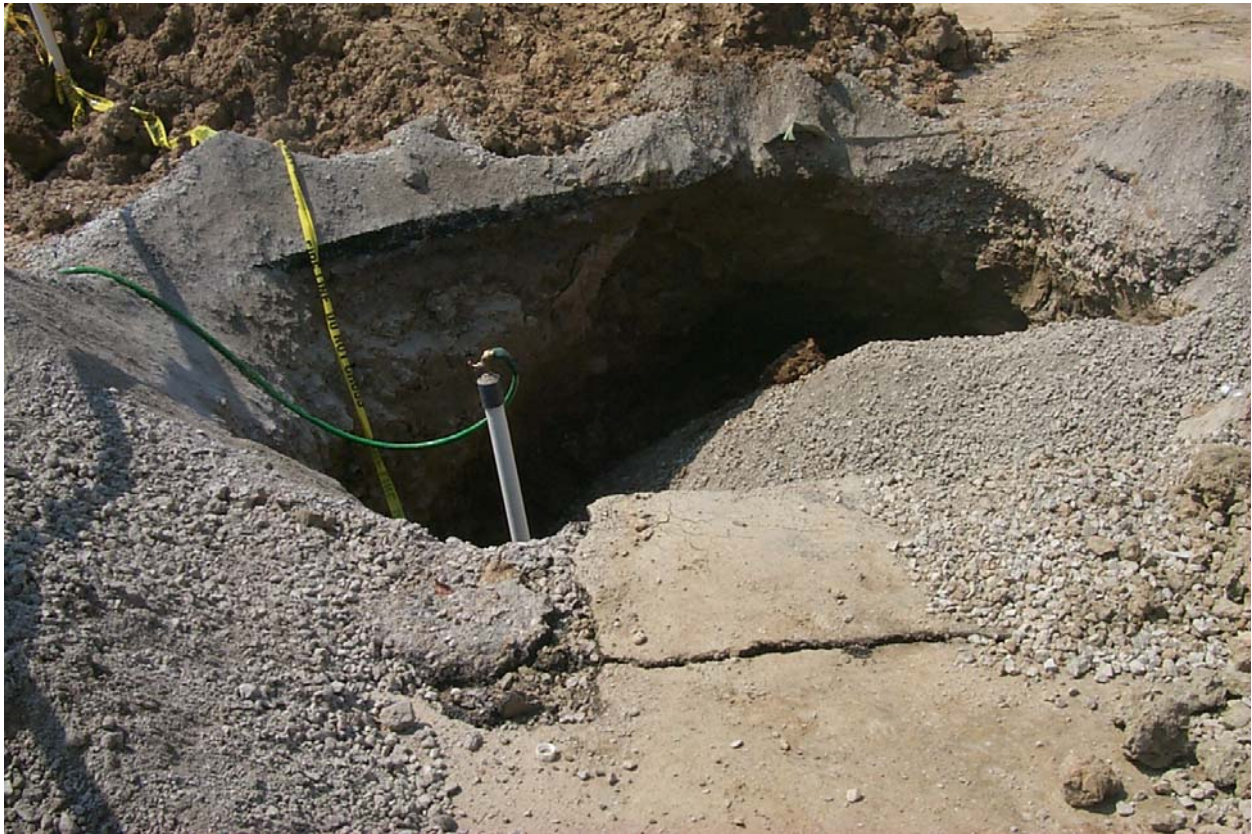
Photograph of Leak No. 1 excavation. Excavation for Leak No. 2 where incident occurred was immediately filled in by the plumbing contractor after decedent had been removed by emergency personnel. This photo was taken the day after the incident.
