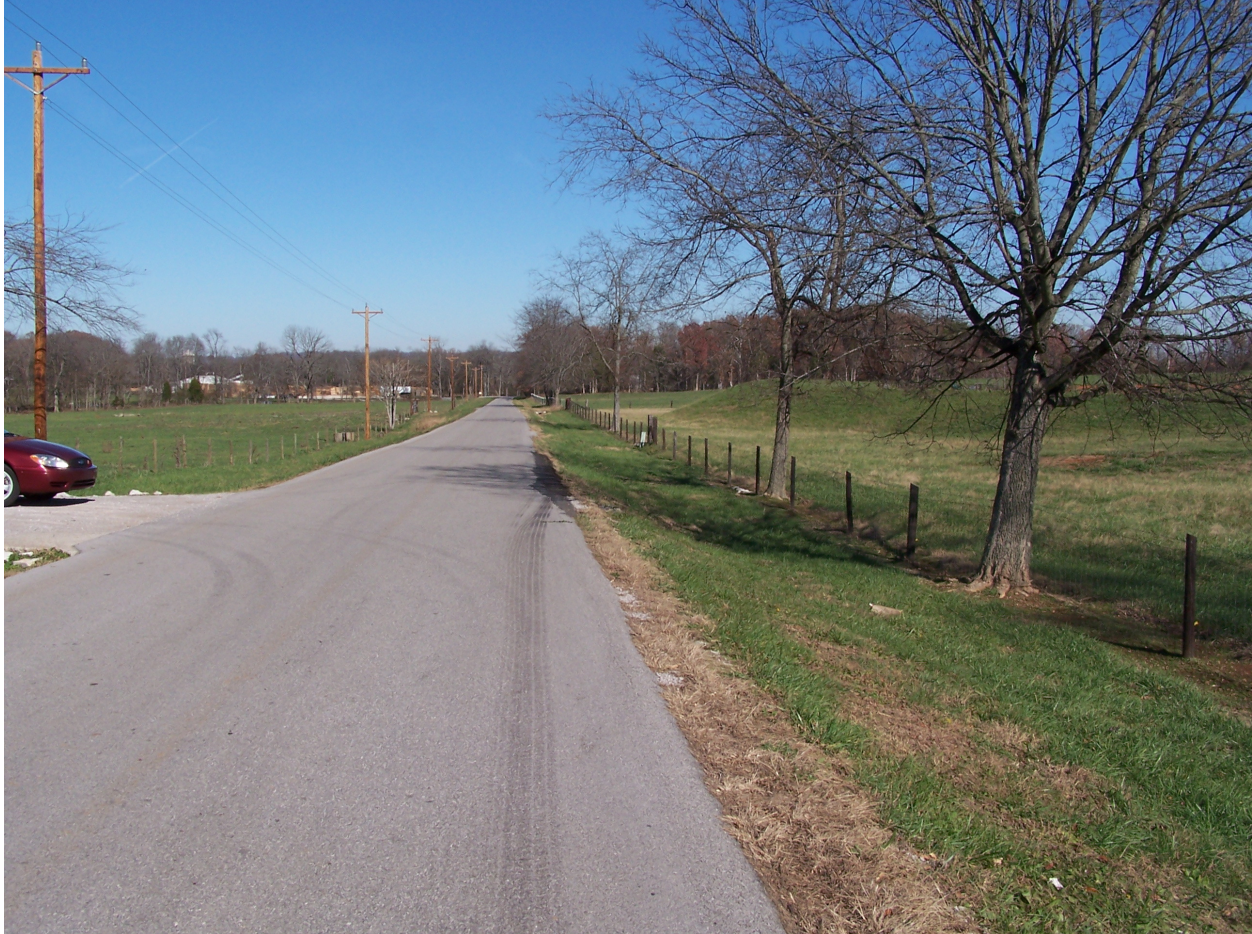
Photograph of county road where a semi-tractor trailer left the pavement and turned over. Grade is steeper than it appears in this photo.
