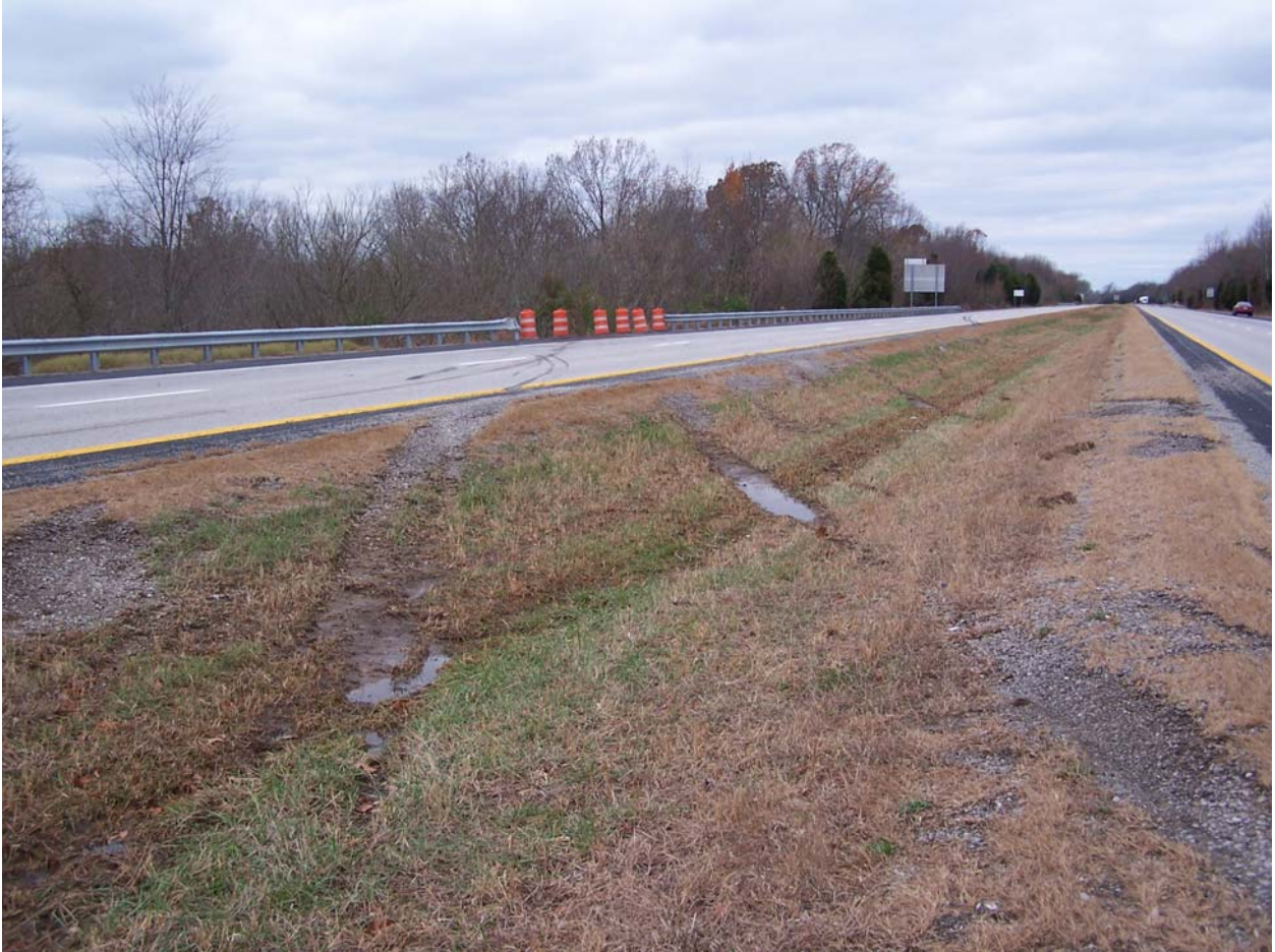
Tire marks from semi-tractor and two trailers crossing parkway median after collision with a cow.
