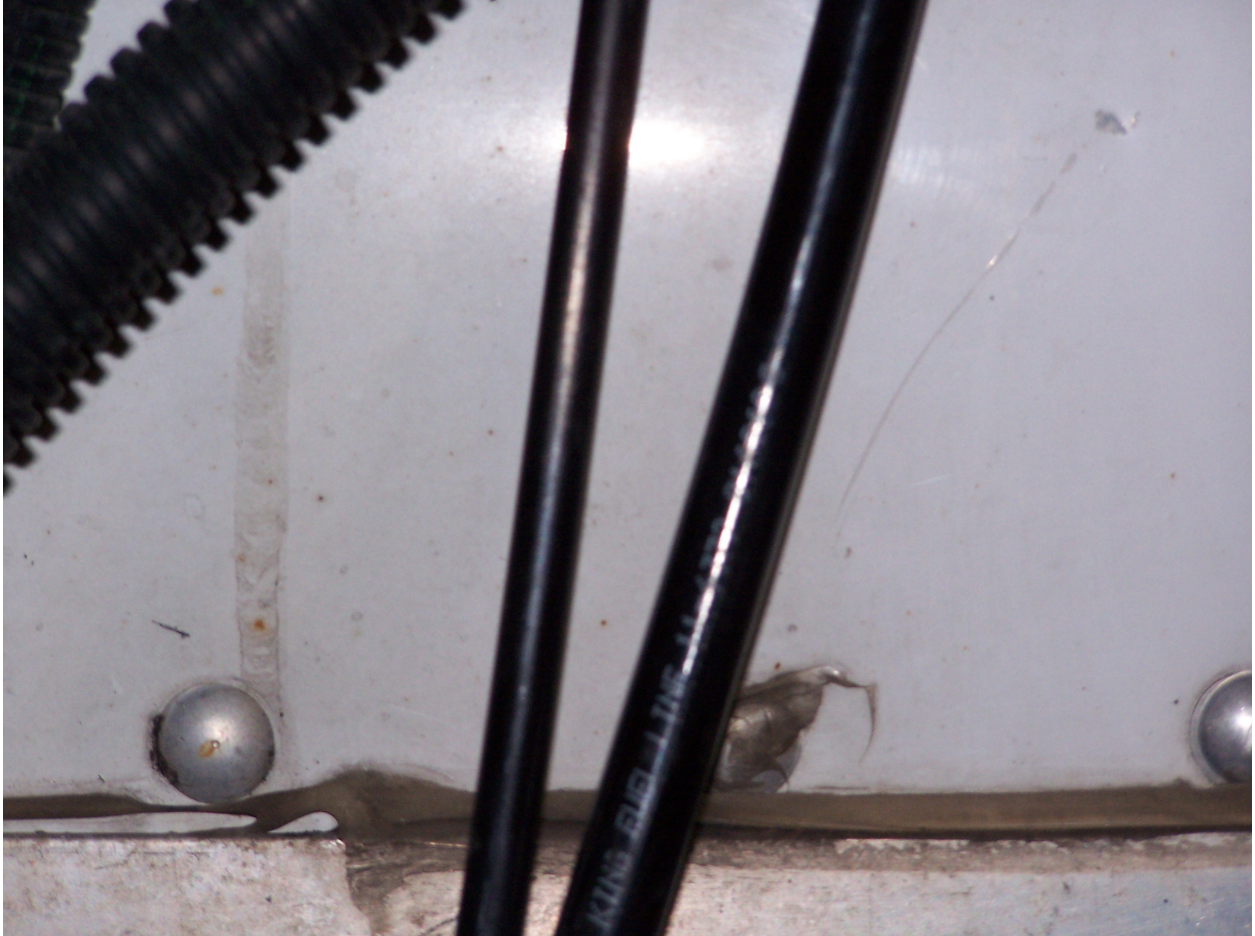
Photograph of the diesel fuel lines on the refrigerated trailer.
