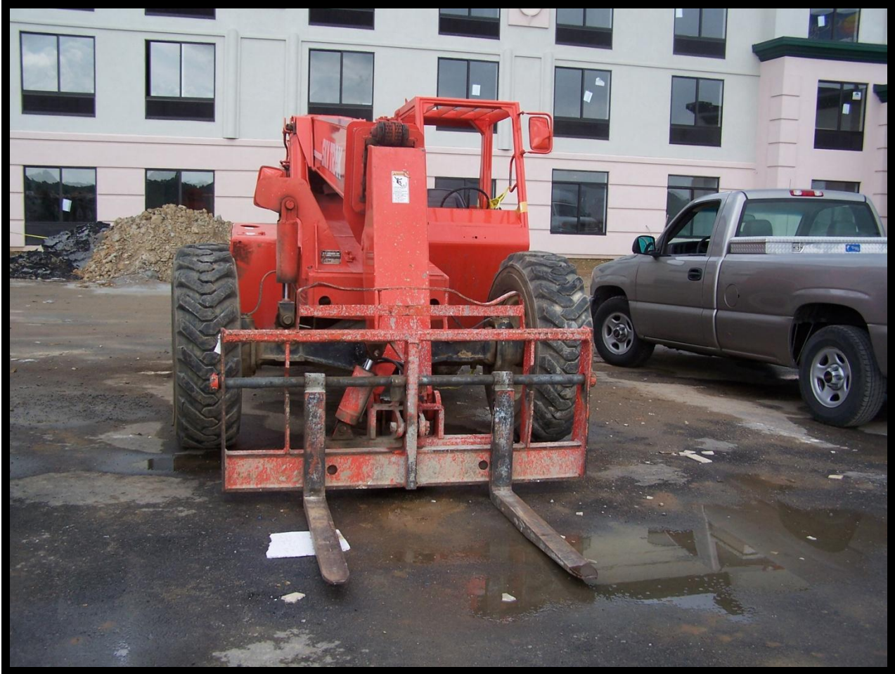
Photograph of forklift used to lift construction box. Photograph property of KY FACE program.
