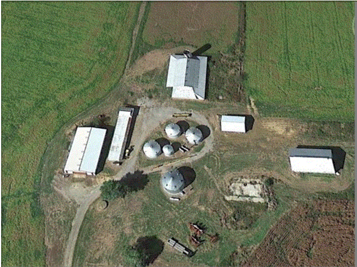
Photo #1 overall view of incident scene
