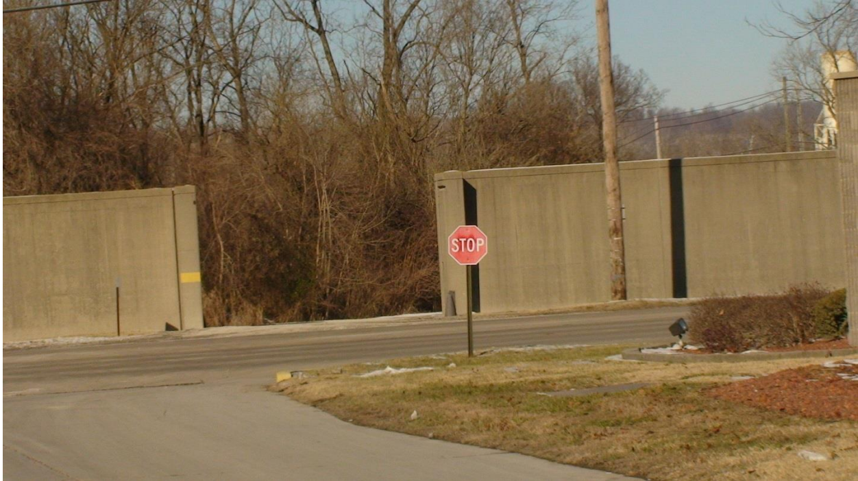
Photograph courtesy of KY OSHA
