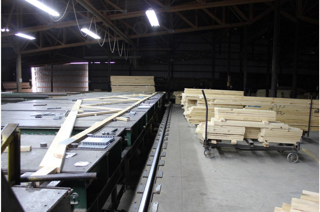
Photo #2 shows the truss being built. Photo courtesy of KY OSHA.
