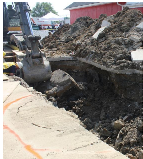
Figure 1. Trench following the rescue efforts.
