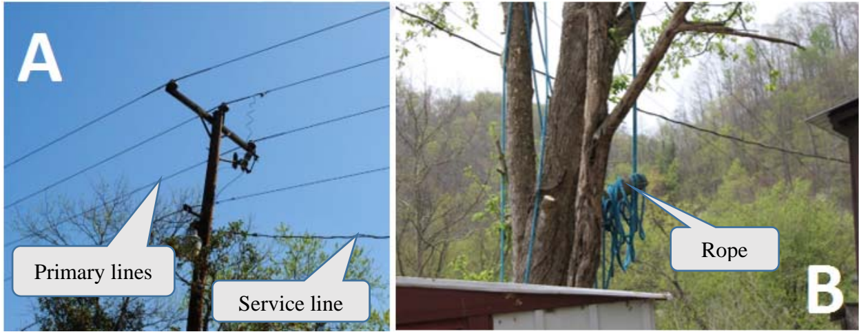
Figure 3. Utility pole that ran power lines behind home (A); climbing rope for victim’s fall arrest system (B).
