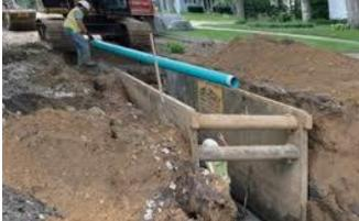
Figure 6. Stock photos of trench shoring (left), trench box (right).
