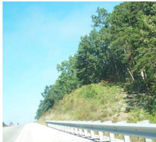
Figure 1. Highway shoulder; approximate location of the collision.
