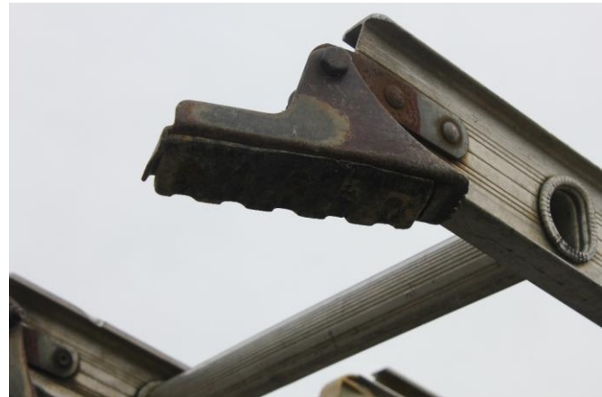
Photo 5: The base of the ladder from which the victim fell. (photo courtesy of KY OSHA)
