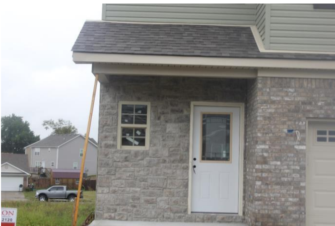
Photo 1: Porch area from which the victim fell (photo courtesy of KY OSHA).
