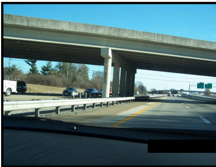
Photo 2. Street level view of the incident scene. Photo property of KY FACE.
