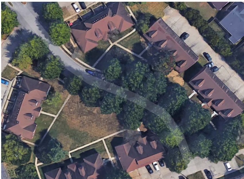
Photo 2: Overhead view of the worksite. All townhouses featured in photo were demolished at the time of the incident. Photo courtesy of Google Maps.
