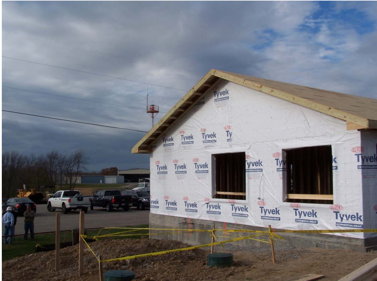
The fall took place from this structure. Photograph property of KY FACE Program
