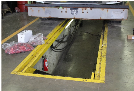
Figure 5. View of the pit from above.
