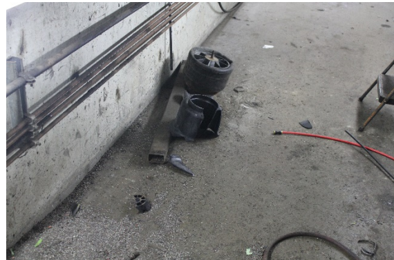
Figure 1. Left side air spring after the explosion.
