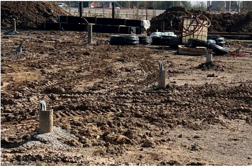
Photo 1. Geothermal system pipes (Property of KY FACE)
