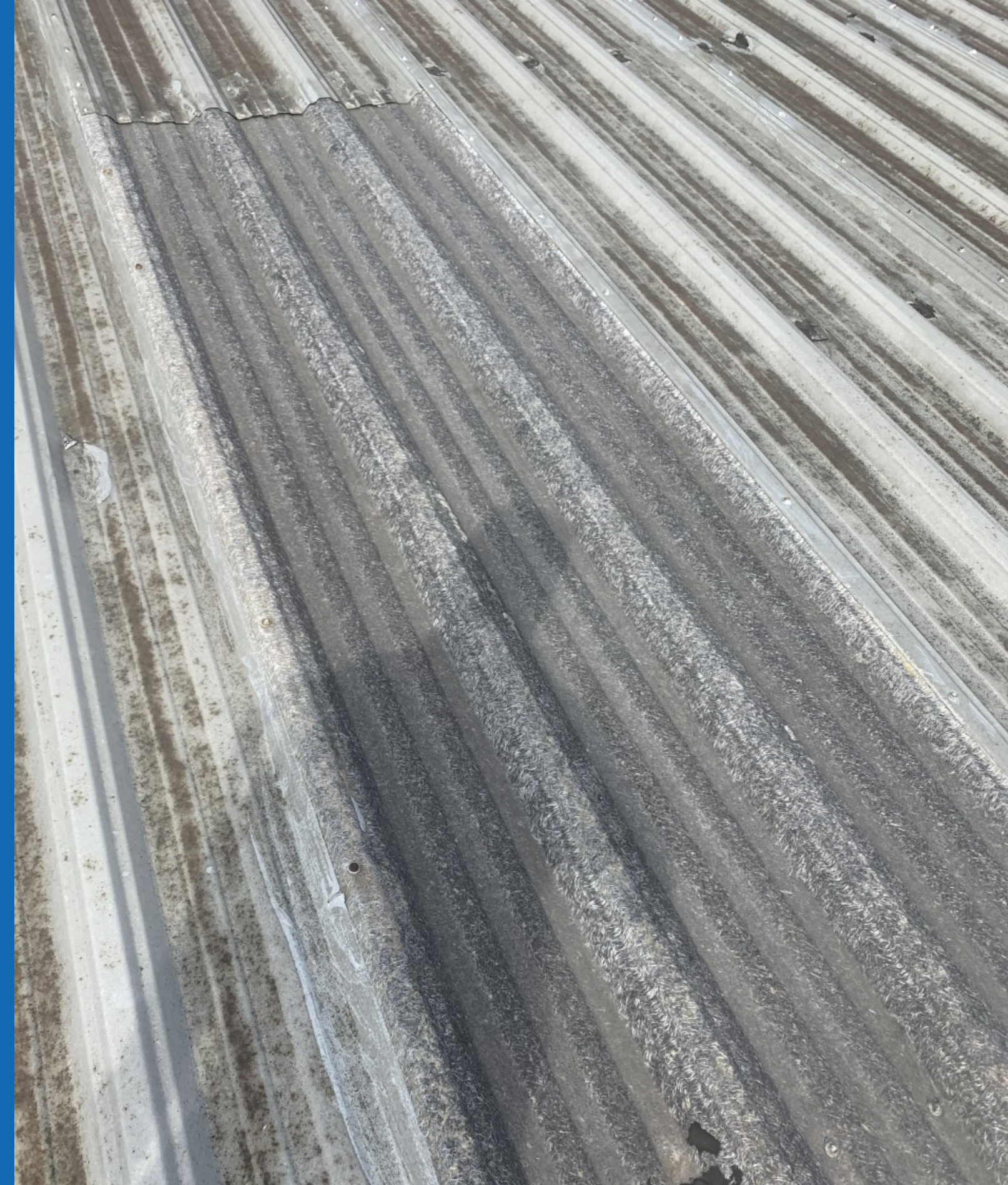
One of the 30 fiberglass skylights present on top of the building where the incident occurred.
