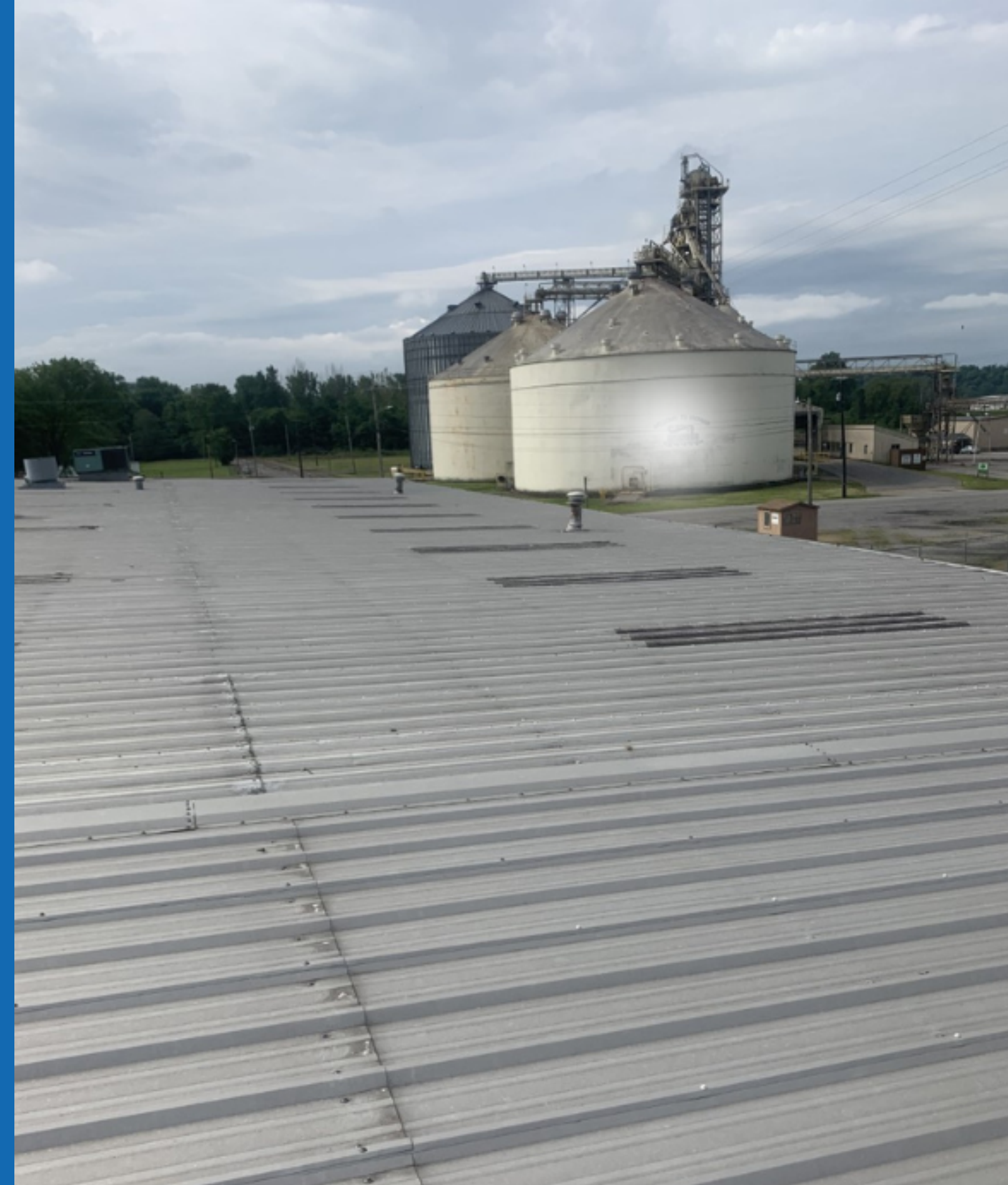
Photo showing metal roof with fiberglass skylights where the incident occurred.
