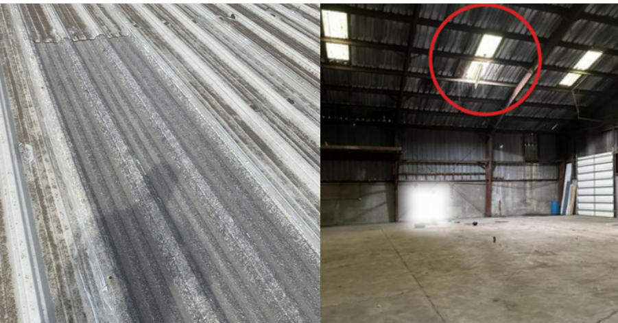
Photo 1: Fiberglass skylight on corrugated metal roof (Case 2).
