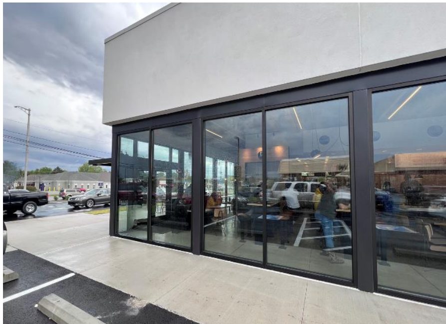
Photo 2. Exterior photo of the building where the incident occurred.
