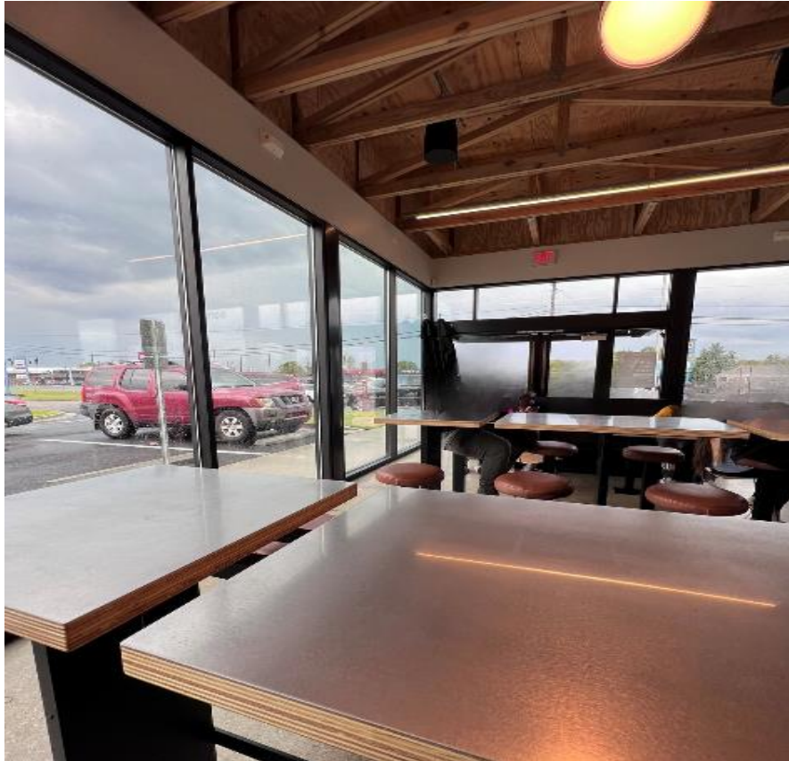
Photo 3. Interior photo of the location where the fall occurred (construction now finished). Photo also shows plywood ceiling panels that were being installed by the victim and his co-worker.
