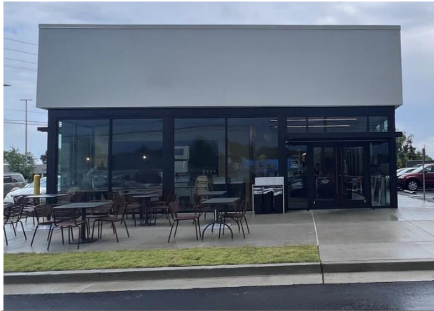
Photo 1. Exterior photo of the building where the incident occurred.
