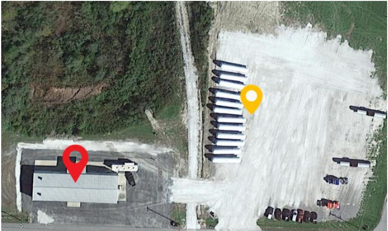
Photo 1. Google Earth photo showing overhead view of the location where the incident occurred. The yellow location marker represents the approximate location of the incident. The red location marker identifies the dual-purpose office and maintenance building occupied by the involved company.
