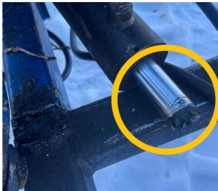
Photo 6. Photo showing post-driver hydraulic arm that was sheared off. Photo provided by involved company.
