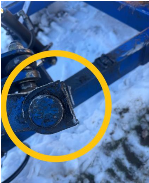
Photo 4. Photo showing post-driver attachment point and point of break. Photo provided by involved company.
