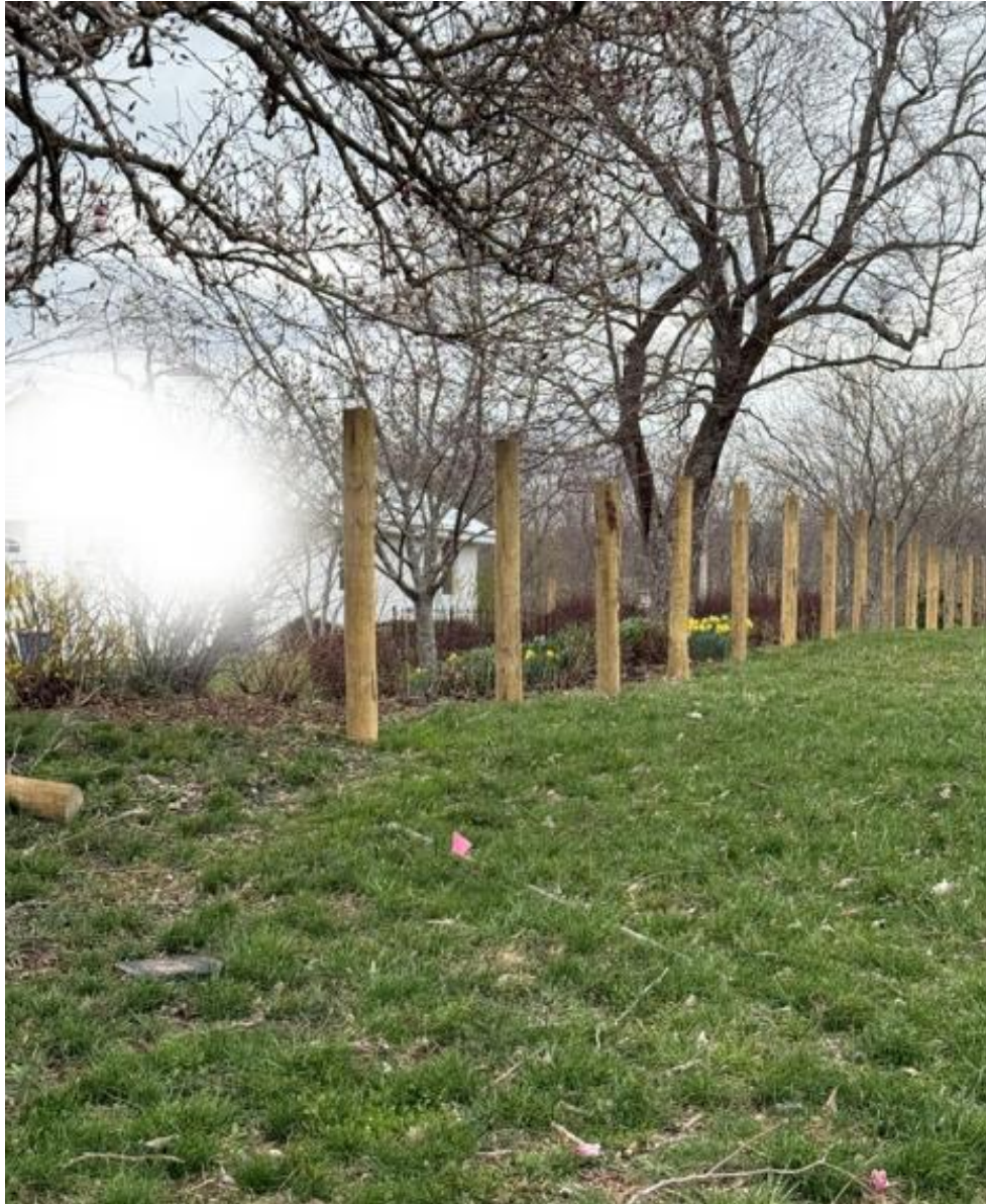
Photo 3. Photo showing posts that were being installed when the incident occurred. Photo property of Kentucky FACE.
