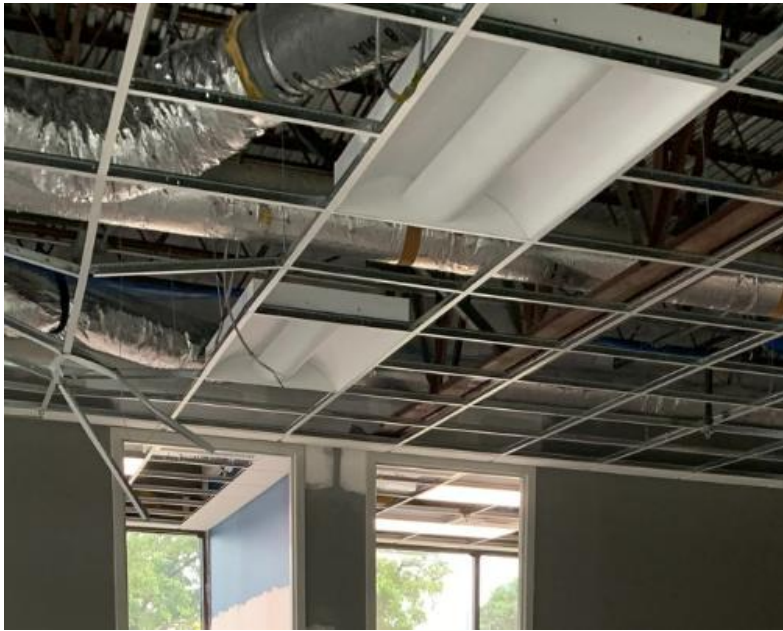
Photo 2: Troffer style lights in the incident. Photo obtained via open records request.
